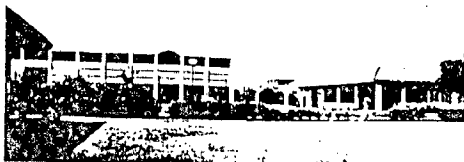
The main compressor plant with the HRD office to the right.
