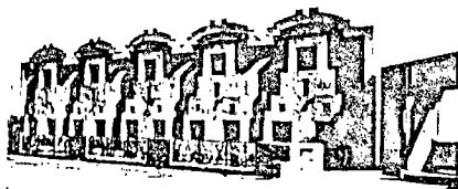
Gentle vault roof and deep recessed windows gives the factory its distinct character.
