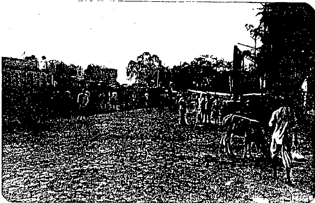
Illu.15) A view of encroachment near recreational park occupying the road space.
