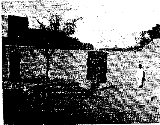
MUD HOUSES SURATGARH TEHSIL GANGANAGAR - Unburnt Brick Walls
