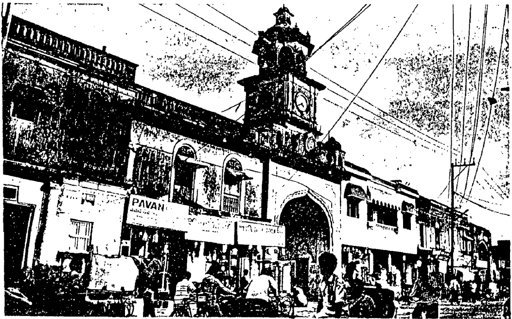
KISHAN PRASAD DEVDI IN DILAPIDATED CONDITION
