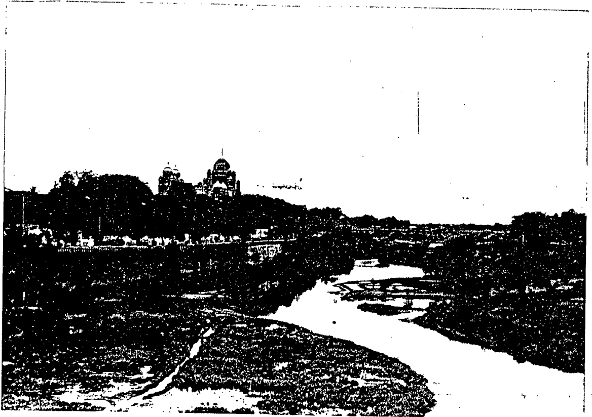
VIEW OF HIGH COURT OVER NAYAPUL BRIDGE .
