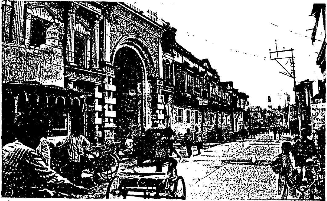
DEVDI EFFECTED IN ROAD WIDENING SCHEME.
