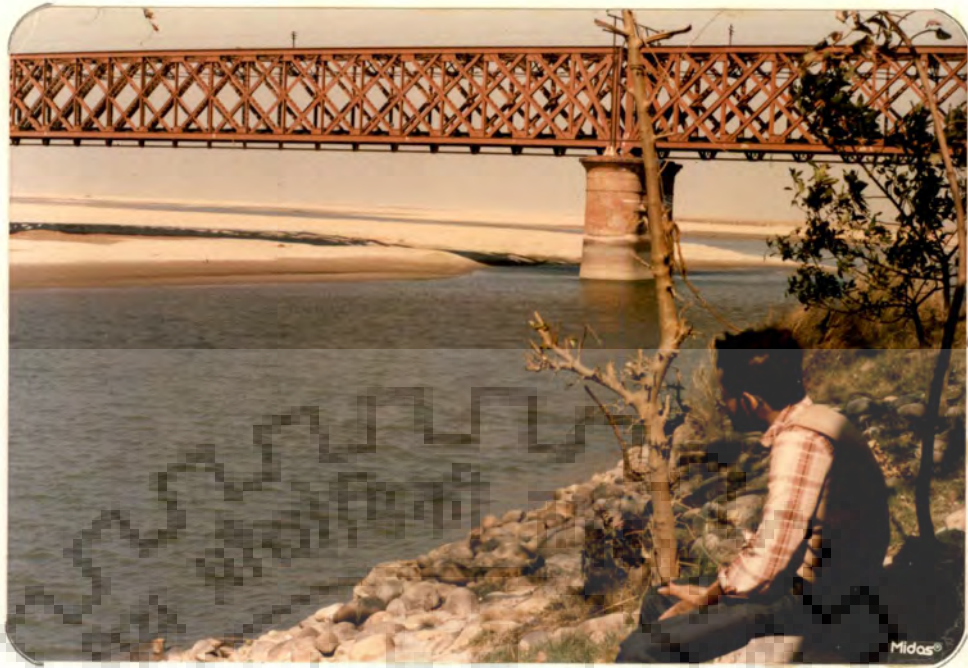
LEAN FLOW CONDITIONS AT BALAWALI
