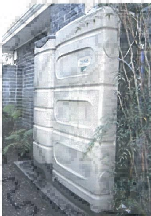
Figure 4.5 Domestic greywater systems by Nubian Water Systems (Oasis GT600)
