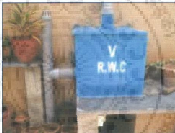
Figure 3.3 Ferro cement filter
