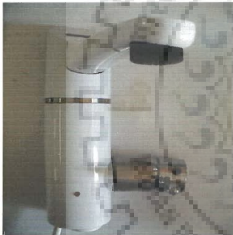
Figure 3.5 Electronic tap (Battery operated), Water saving 60%.
