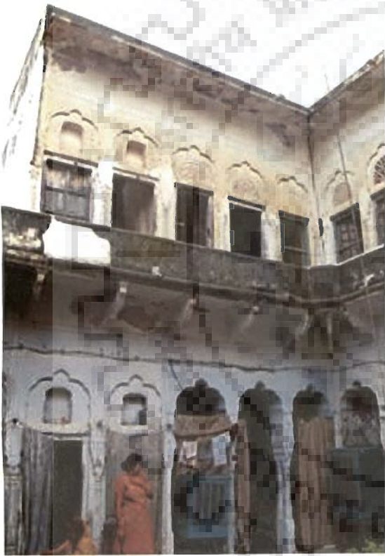
Partly constructed first floor
