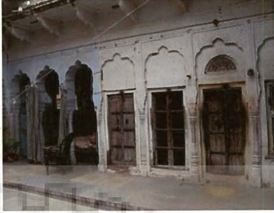
Kitchen, Parinda & Staircase
