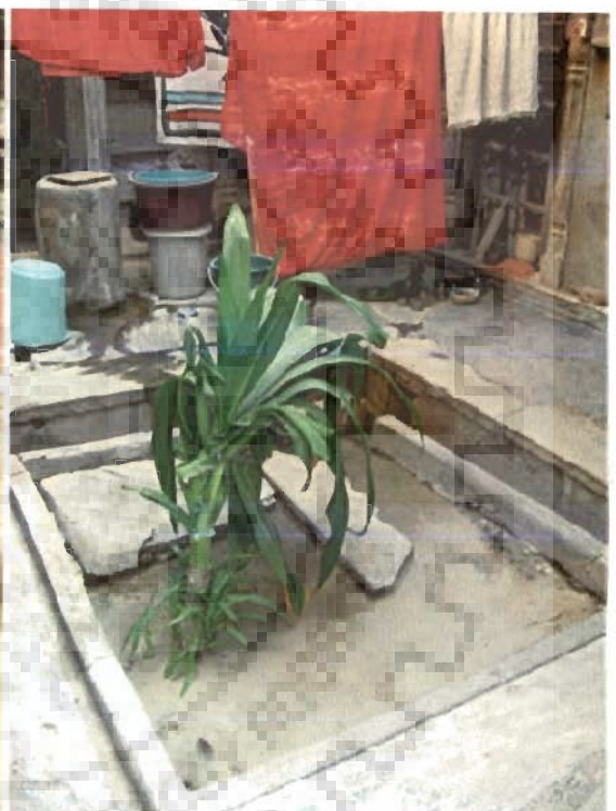
Soft paved inner court
