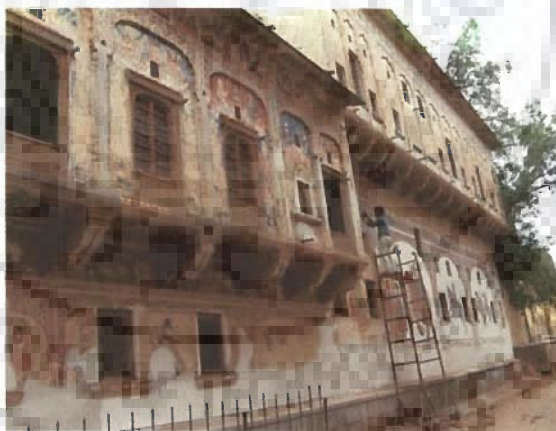
Figure 3.6.2.1 Jharokhas projecting out on wall, help in shading the wall
