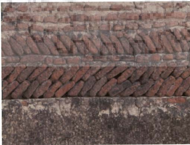
Exposed wall showing brick arrangement
