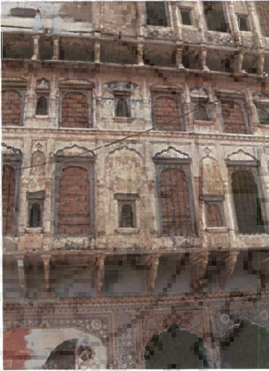
Windows on front facade
