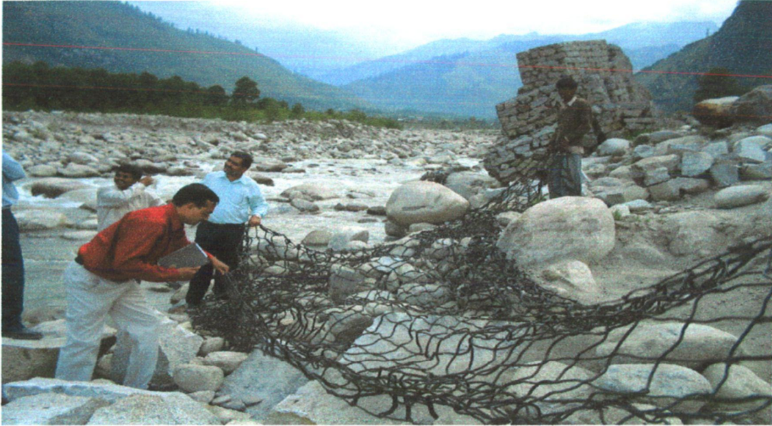
Fig-9.5 Polymer Rope Gabion Box Carried to the River Bed
