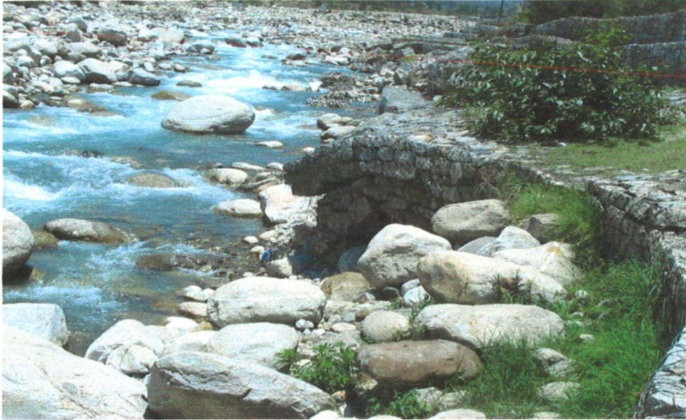
Fig-9.3 Due to Rigidity GI Wire Gabions do not Adhere to Undulation
