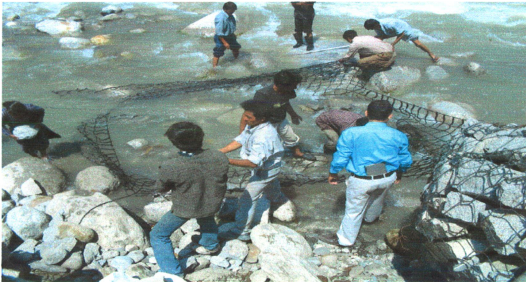
Fig-9.6 Polymer Rope Gabion Box is Anchored
