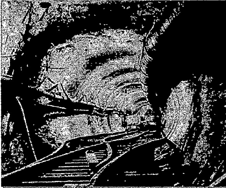
Fig.4.21 Transition from conventional method (drill & blast) section to boring machine tunnel, display difference in quality of hole resulting from two methods. (12)
