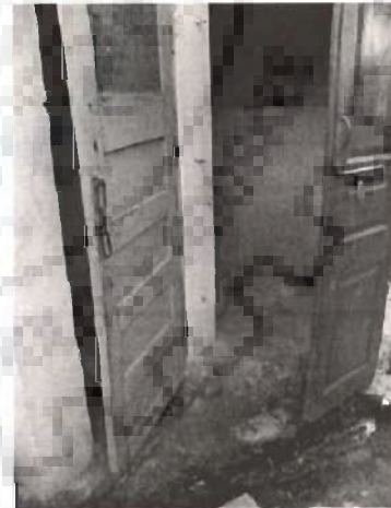
Fig. 5.78 Wooden door of a bathing space with a small chain hanging outside for pulling the door outwards and bolting it.
