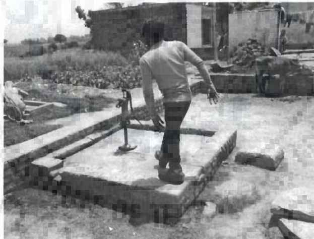
Fig. 5.35 Typical community Hand pump space with a square plinth around it in the study area.
