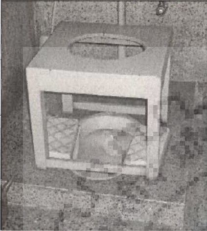
Fig. 2.14 Wooden toilet seat placed over squat toilet
