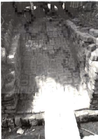
Fig. 5.48 Brick paved ramp used by Vikas for reaching the toilet facility.
