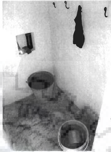
Fig. 5.80 Niche for keeping bathing accessories at a low height for easy access
