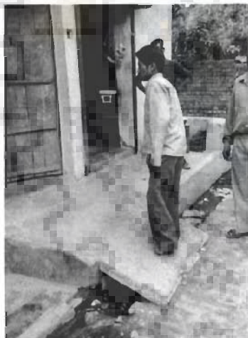
Fig. 5.24 Pankaj using a ramped approach to climb threshold level to his house.
