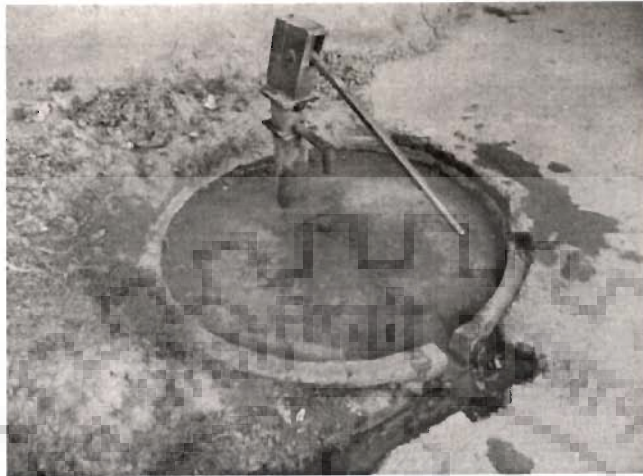
Fig. 5.36 Typical community Hand pump space with a leveled approach from one side in the study area.
