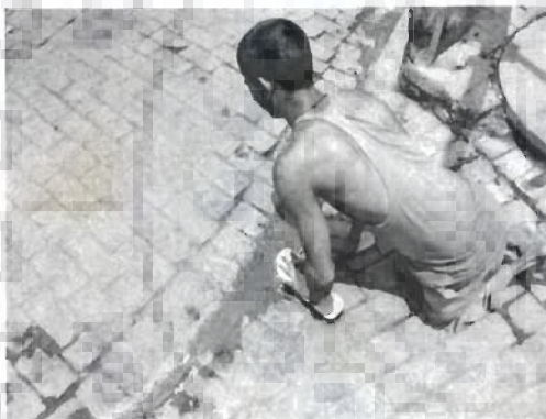
Fig. 5.9 Momin Ahmed uses bathroom slippers as an aid to prevent his hands getting bruised.
