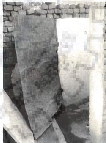
Fig. 5.57 Toilet door made out of scrap iron.
