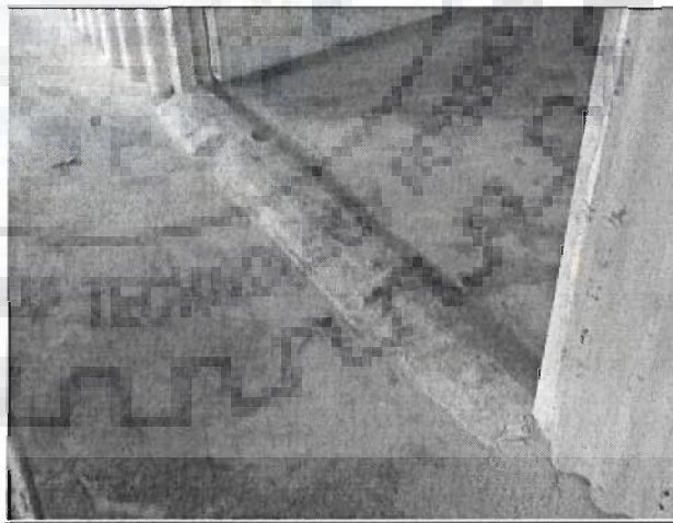
Fig. 2.17 Rounded Threshold for bathing space, surmountable by wheelchair
