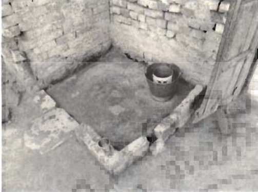
Fig. 5.67 Cemented platform as bathing space near the entrance of the house.
