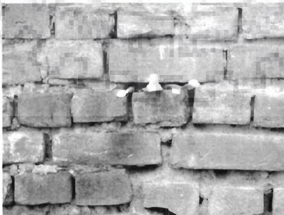
Fig. 5.85(c) Grooves in the wall being used as storage space
