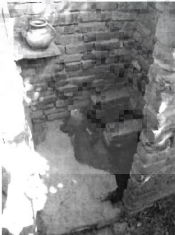
Fig. 5.52 Side approach for a dry squat toilet with two brick platforms for squatting.
