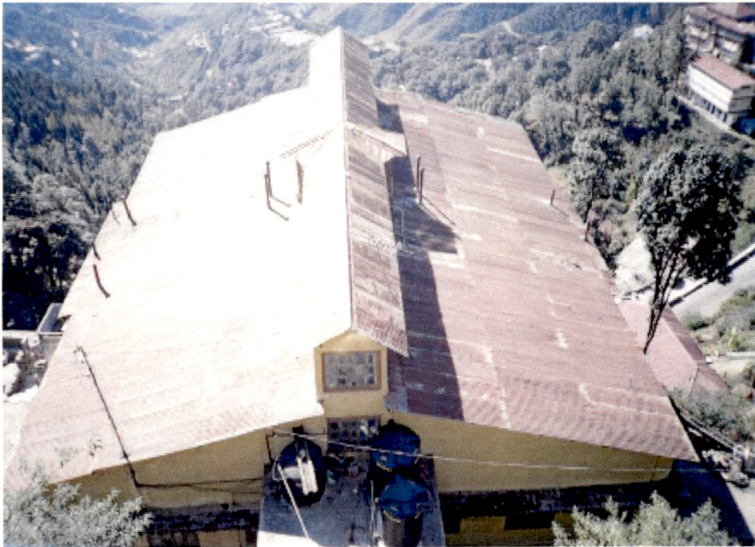
FIG. 6.7 : AERIAL VIEW OF STELLA COTTAGE
