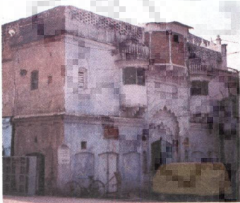
Figure 4.11 Jharokha induces forced air
