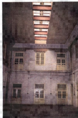
Figure 4.12 Skylight for light and ventilation
