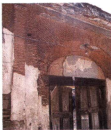
Figure 3.8 Thick Masonry of Lakhauri bricks
