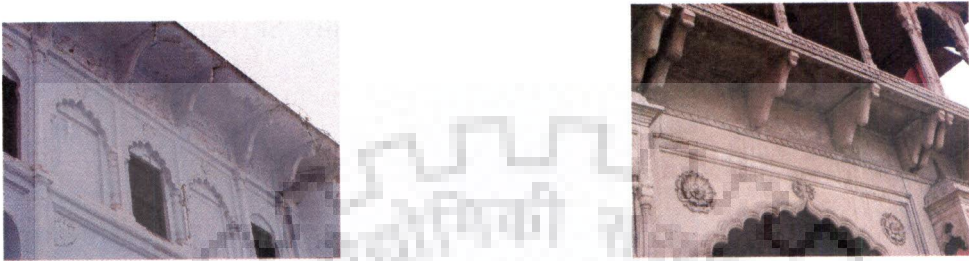
Figure 4.13 Overhangs and projections provides shade from direct solar radiation
