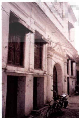
Figure 5.18 Front view from the street
