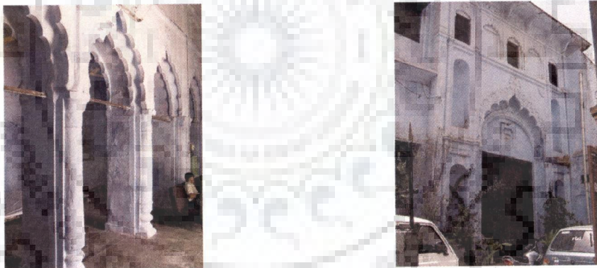
Figure 4.7 Massive walls increases time lag
