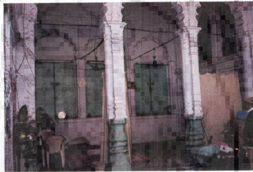
Figure 5.11 Double Height of Imambara
