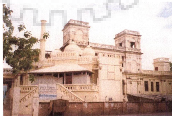
Figure 5.2 Northwest corner of the building
