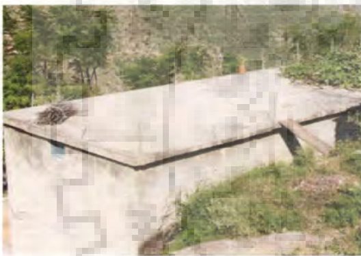
(a) RCC roof over brick wall
