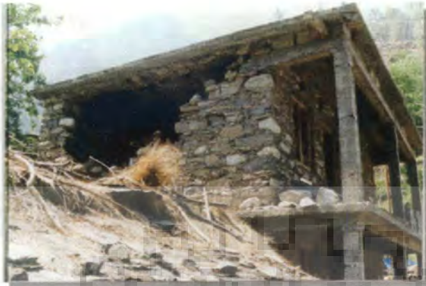
(a) Collapse of slate and stone masonry wall with poorly designed RCC construction
