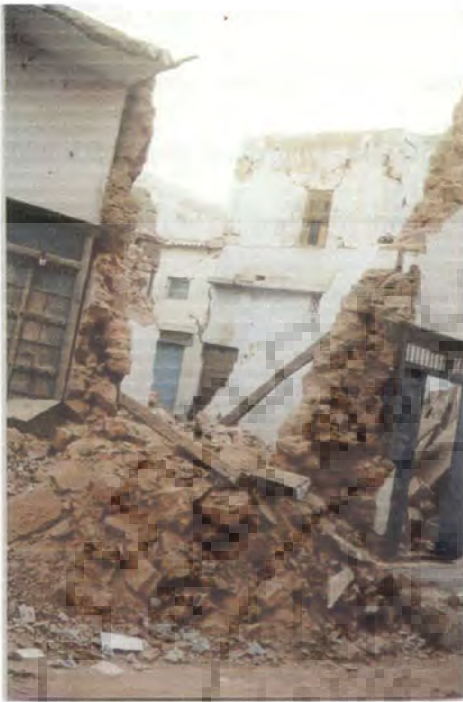
Figure 3.22: Damage to random rubble stone masonry
