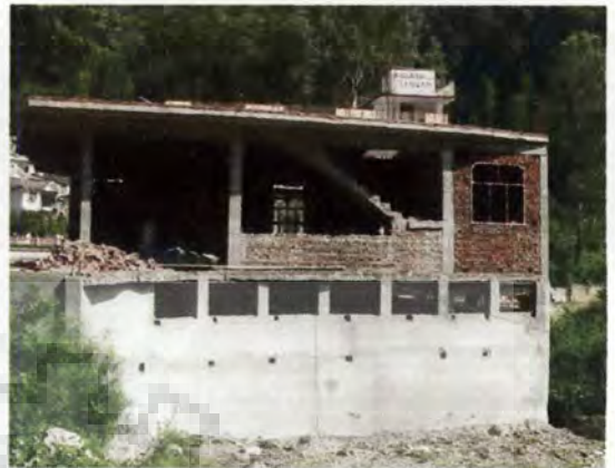
(b) Brick wall with RC frame in Tapowan
