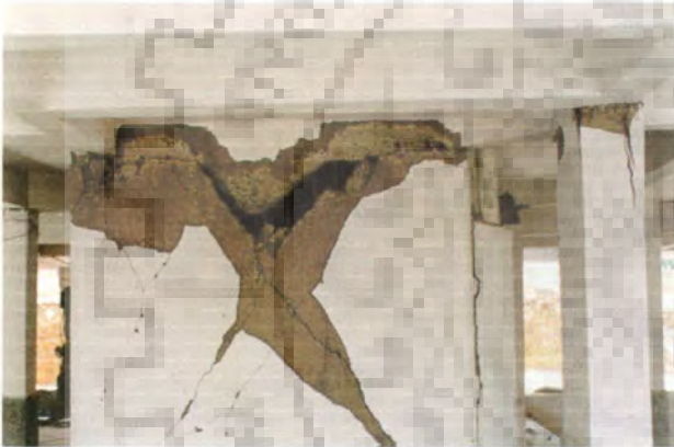
(a) Damage to RC framed railway station during Gujarat Earthquake, 2001
