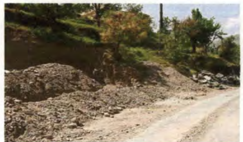
Figure 9: Landslide on access to Odada
