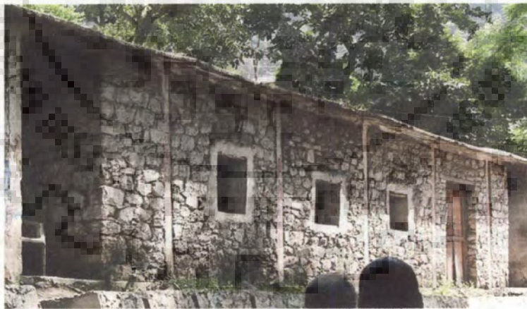
Figure 3.23: Stone in cement and sand mortar
