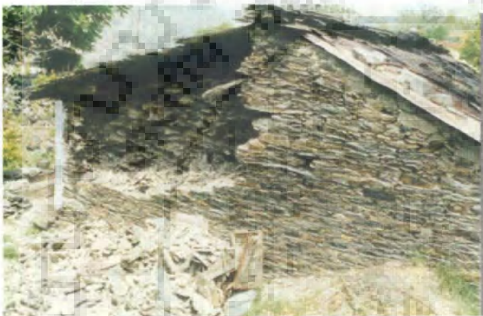
Figure 3.20: Damage to stone and slate masonry during Chamoli earthquake
