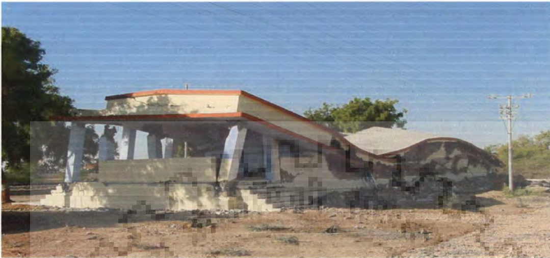
(a) Damage to RC framed railway station during Gujarat Earthquake, 2001
