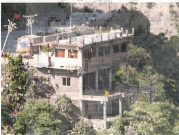
(a) Rc Frame structure near Tapowan
