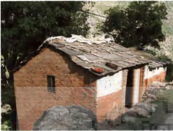
Figure 3.26: Earth walls in Narendranagar block
