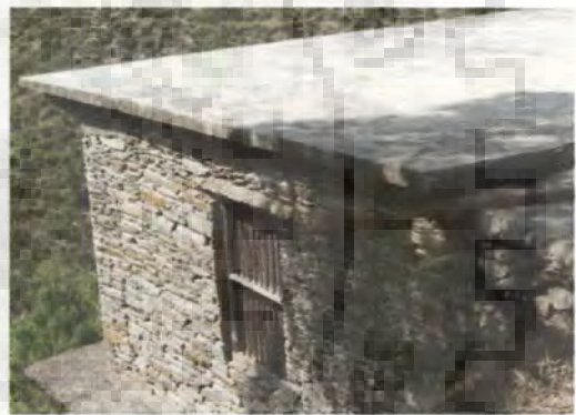
(b) RCC roof over stone wall
