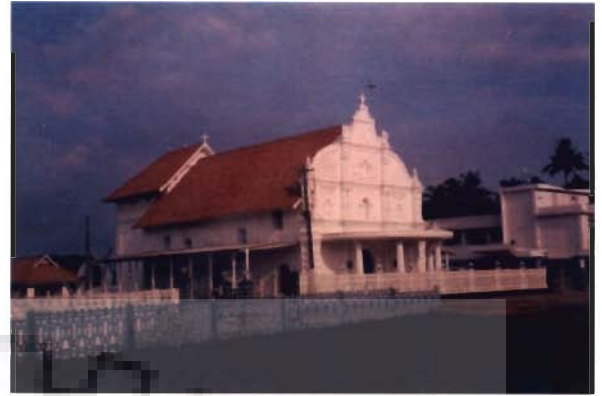
Photo 3.26 Sloping Hykala roof of Kothamangalam cheriya palli
