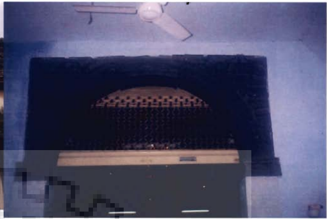
Photo 4.32 Single piece stone arch in Kottayam Valiya palli
