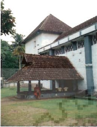
Photo 3.31 Mukha-mandapam of Chenganoor church on Northern side
