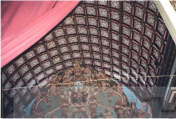
Photo 4.19 Vault built of wood in Chembakkulam church
