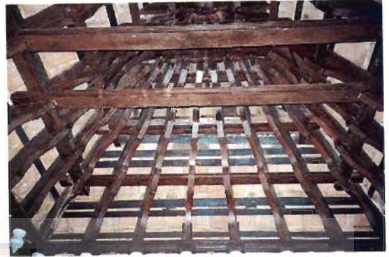
Photo 4.38 Carved roof of Mukhamandapam in Chenganoor church
