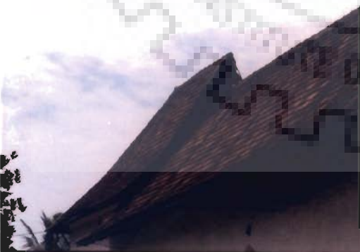
Photo 4.29 Madbaha roof projected just a little in Purakkad church
