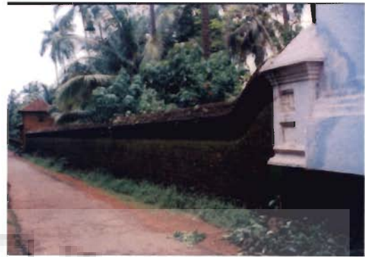
Photo 3.32 High compound wall in Arthaat church
