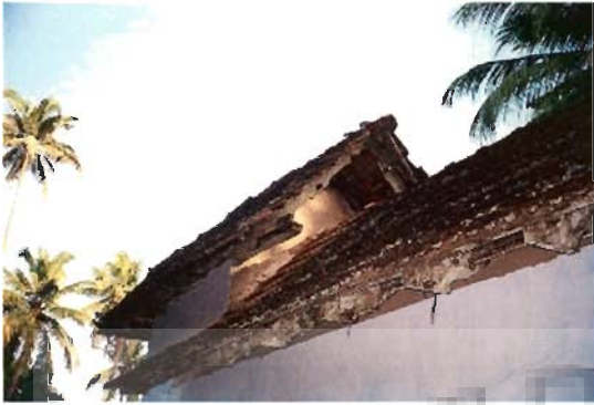
Photo 3.79 Madbaha roof higher than Hykala roof in Pallippuram kurishu palli
