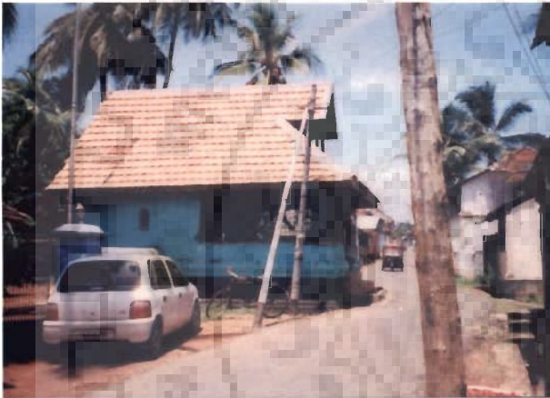
Photo 4.81 Present view of Ambala-palli with the wooden trellis work removed ...
