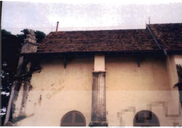
Photo 4.31 Madbaha roof lower than Hykala roof in St. Francis church
