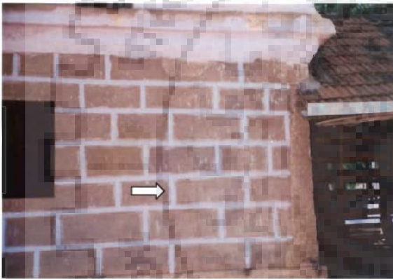
Photo 3.105 Granite pillars embedded inside the wall
