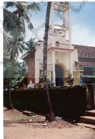
Photo 4.78 Existing part (Madbaha) of old Eanammaavu church
