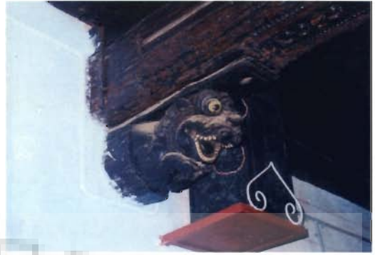
Photo 3.62 Balcony bracket in Kottapadi church
