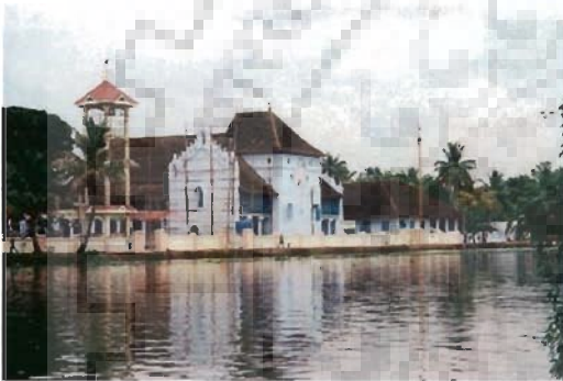
Photo 3.51 Chembakkulam church, flag post can be seen on right side
