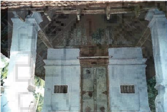
Photo 3.93 Wooden partition used in Mattam kurishu palli
