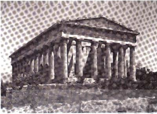
Photo 2.7 A Greek temple with decorated exterior columns
