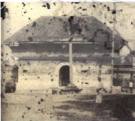
Photo 3.35 Original Padi-ppura in Kanjoor church (now demolished)
