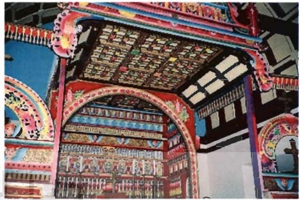
Photo 4.14 Second roof under vault in Chenganoor church
