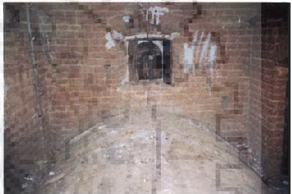
Photo 4.22 Space over the vault in Kunnumkulam church
