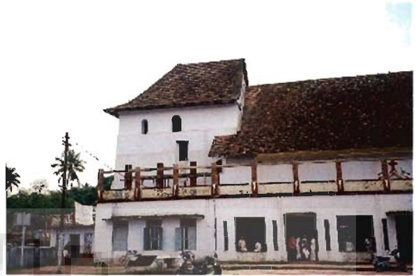
Photo 2.26 High roof for Madbaha (Thora) in Muttam church
