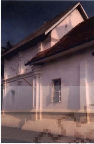
Photo 3.25 Kothamangalam Valiya palli with Madbaha higher than Hykala roof
