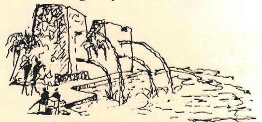
(g) Water getting out of a Stone Wall
