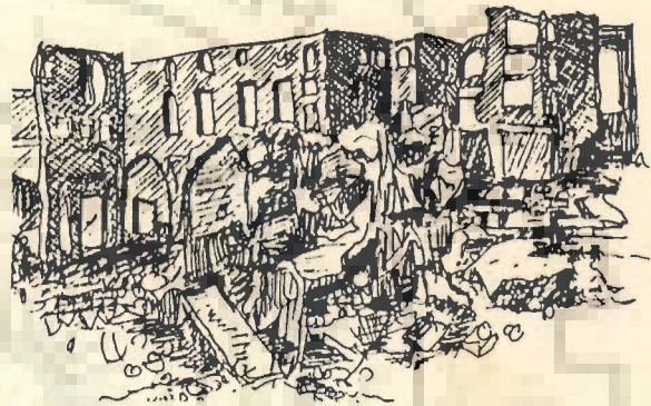
Fig.3.32 : Dilapidated building old - core B.Lengeh
