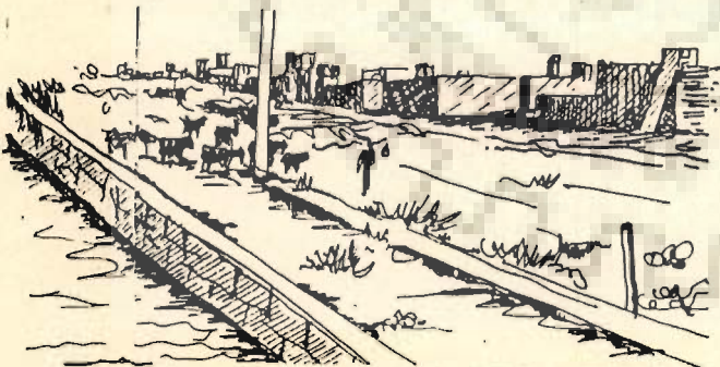
e) Directing Flood to the "Berkeh" by Building Low Stone Walls
