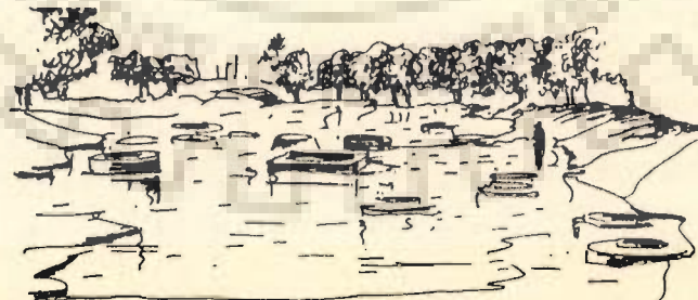
Digging Wells in the bed of Floodway To Take Water to the Under Ground Water Water table - Bandar Lengeh
