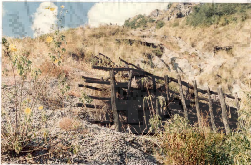
PHOTOGRAPH 3.8- Crib structures filled with brushwood on moderate slopes.
