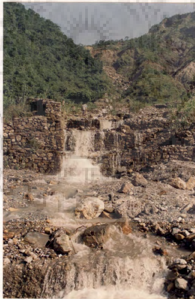
PHOTOGRAPH 3.4- Gabion structures in main drainage channel of Jhandoo-Nala watershed.
