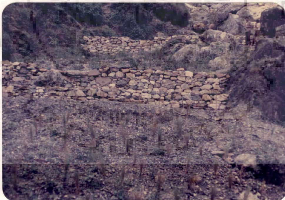
PHOTOGRAPH 3.6- Grass clumps planted between the loose rock filled check dams.
