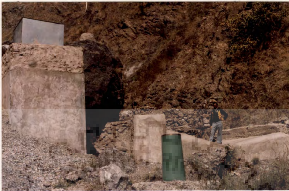
PHOTOGRAPH 3.3- A view of the trapezoidal flume constructed at Jhandoo-Nala.
