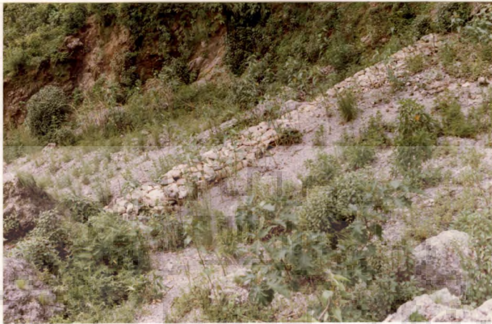
PHOTOGRAPH 3.5- A view of vegetation planted on the banks and bed of main drainage channel.
