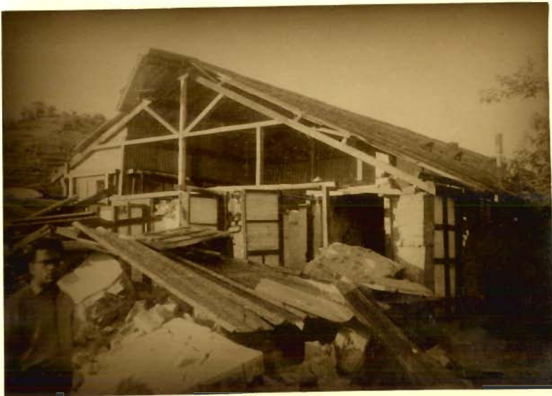
FIG. 3-3. PHOTOGRAPHS SHOWING TYPICAL DAMAGE AT KOYNA DECEMBER 11, 1967 EARTHQUAKE
