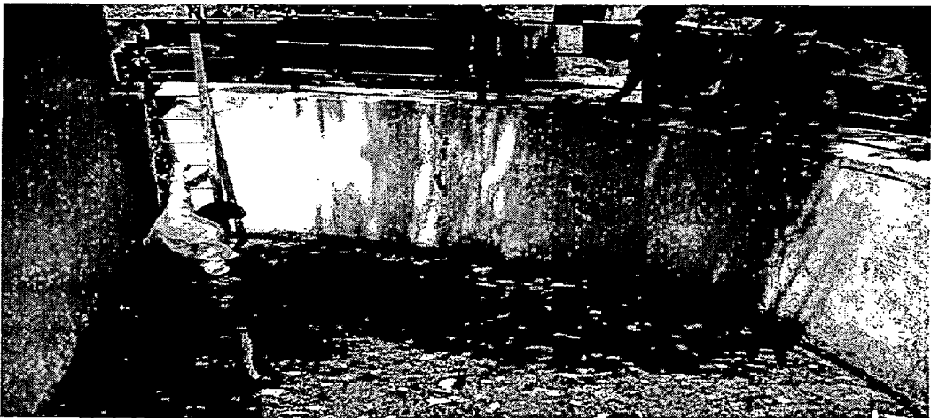
Fig.2.9. Khanjarpur Sewage Pumping Station, Roorkee.
