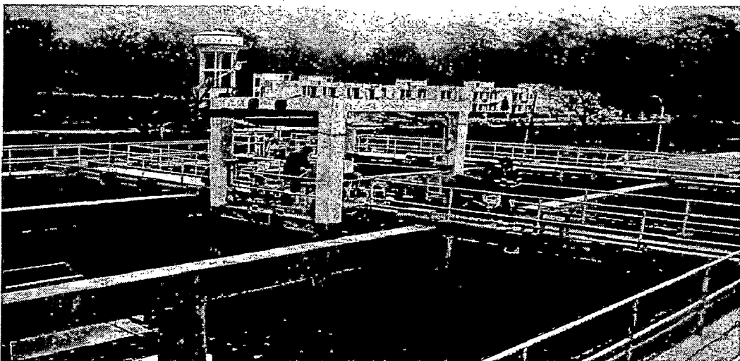
Fig 2.10. Rishikesh sewage plant.
