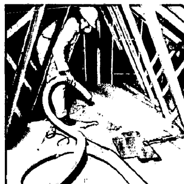
Spraying in cellulose loft insulation Source: © Excel Industries
