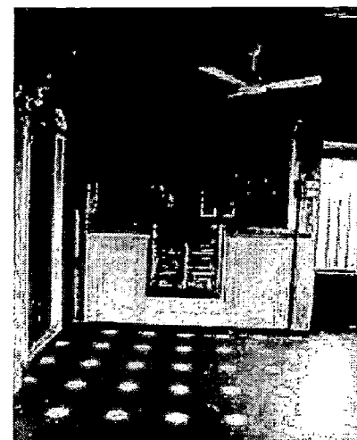
Figure 32 Flooring re-laid matching with previous flooring
