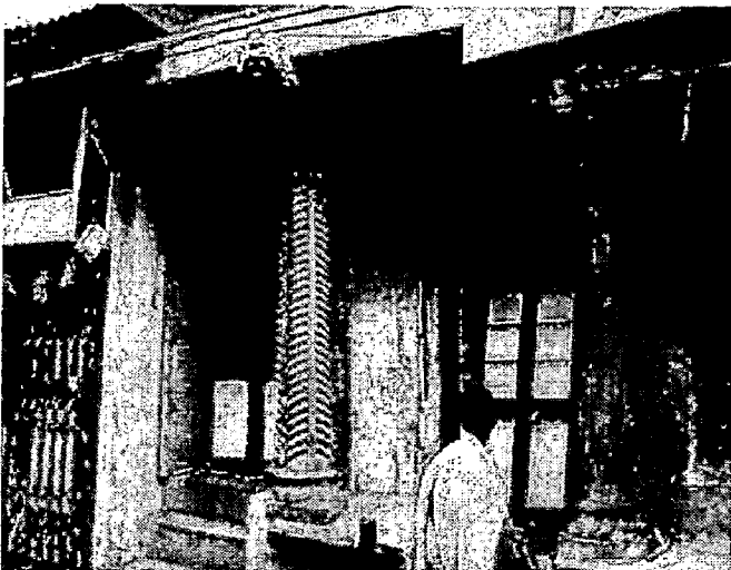
Figure 59 Wooden Columns, Pol Houses Ahmedabad
