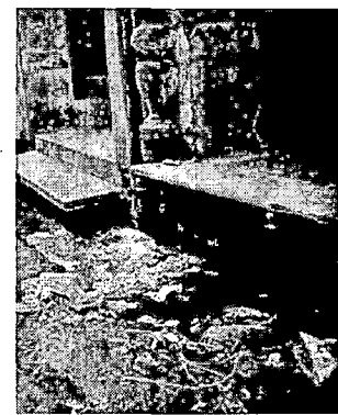
Figure 5.7.6.4 Clogged drains at Katra Ahluwalia (Source: By Author)
