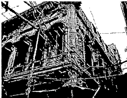
Electric Wires Degrading Heritage of City
