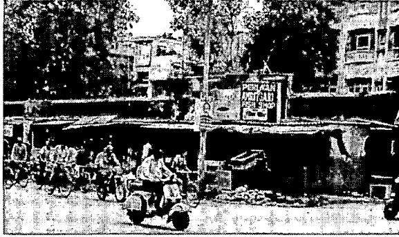
Figure 5.7.2.2 Old Wall of Walled City behind temporary shops. (Source: By Author)
