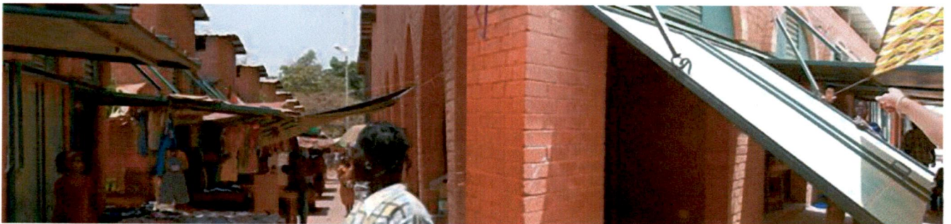
Figure 31 Two-Hinged Doors (Source: AKDN)
