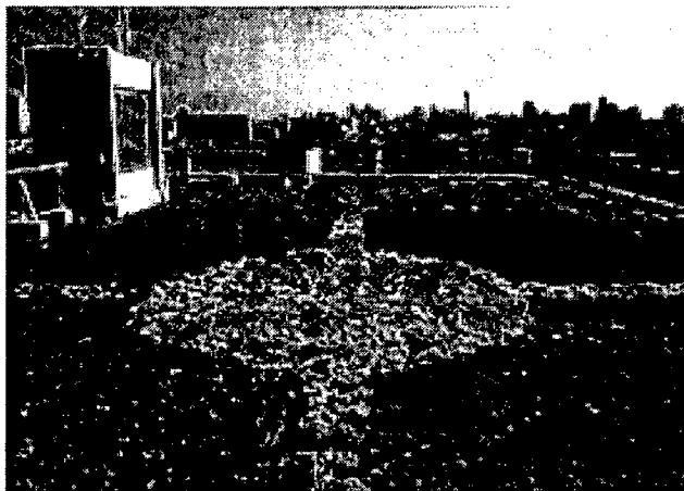
Figure 31 Extensive Green Roof
