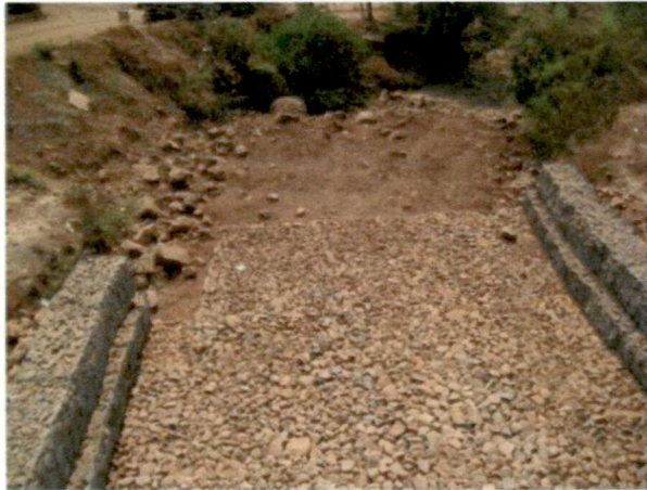
Nallah gabion channelization at Dasve.
