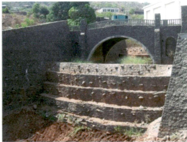
Nallah retaining wall channelization at Dasve.
