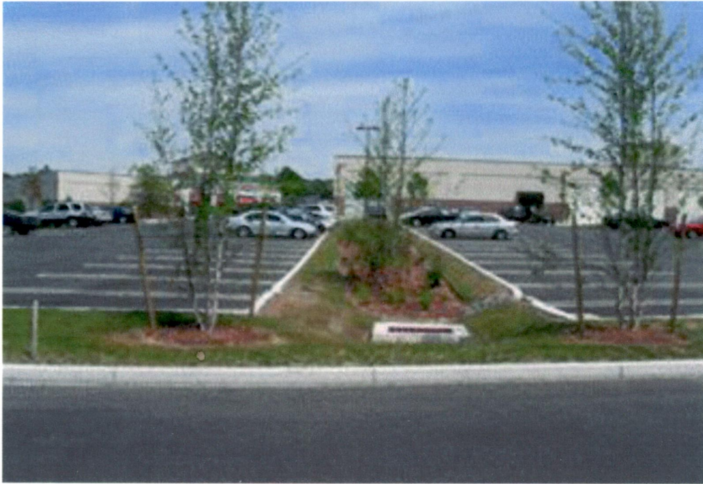
Figure 20 bioretention median in a parking lot
