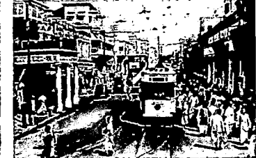
6. Early development concentrated around tram line, Kolkata, India
