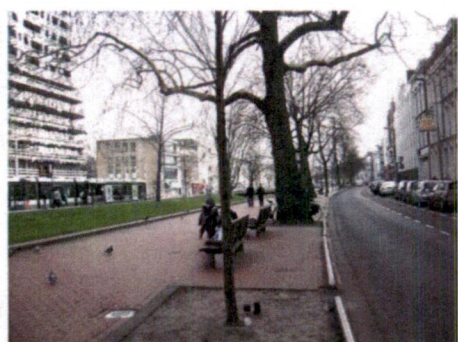
4. Limiting width of vehicular carriageway and introducing central pedestrian walkway & green area- Rotterdam, Netherlands (05-03-2012)
