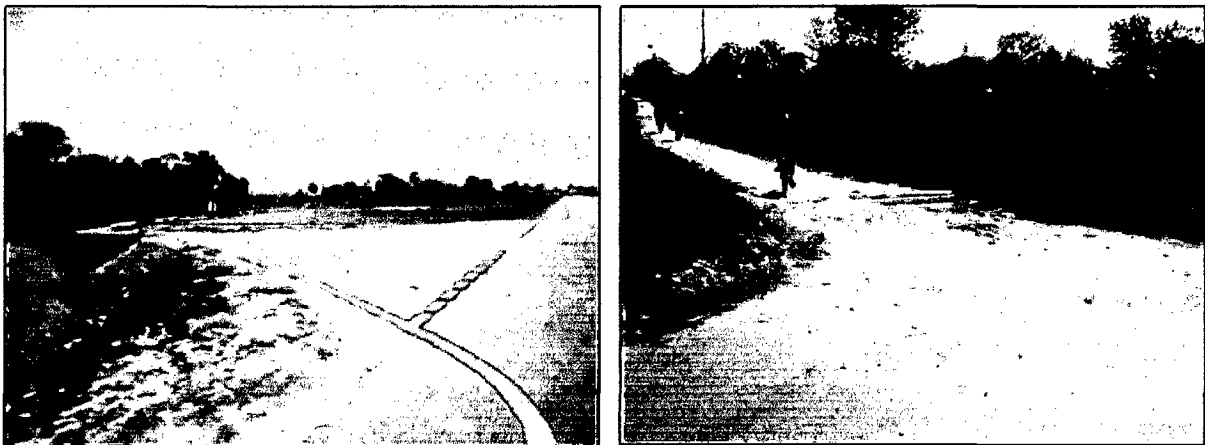
Figure 115: Picture showing Minor Junctions as Provided during Four Laning
