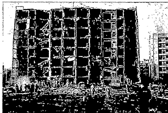
Figure 15: Exterior envelope failure because of direct air-blast effects.
