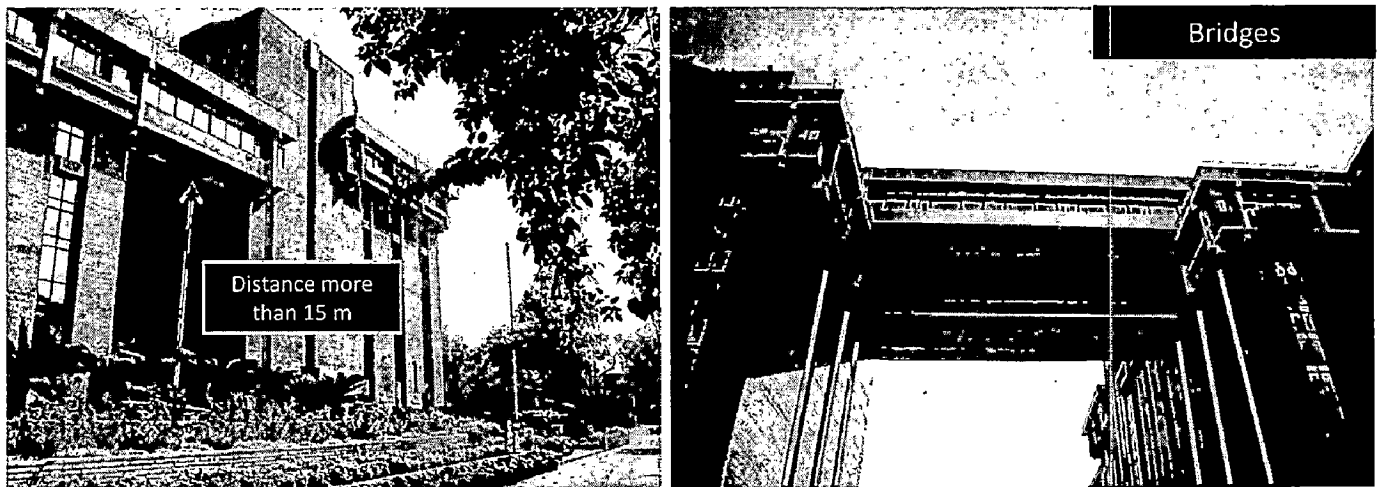
Figure 142: Stand-off distance of bridge is greater than 15m from the ground.
