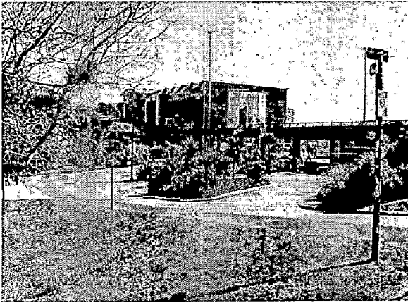
Figure 61: Approach road to the building is parallel to the building
