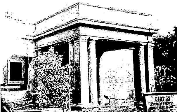
Illus. 9 Seismic Retrofit of historic masonry load bearing structure in Lutyen's Delhi
