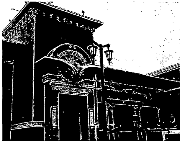
Illus. 14 The cheese Cake factory - FRP was used in all cornice, columns, medallions and finials (DEC)
