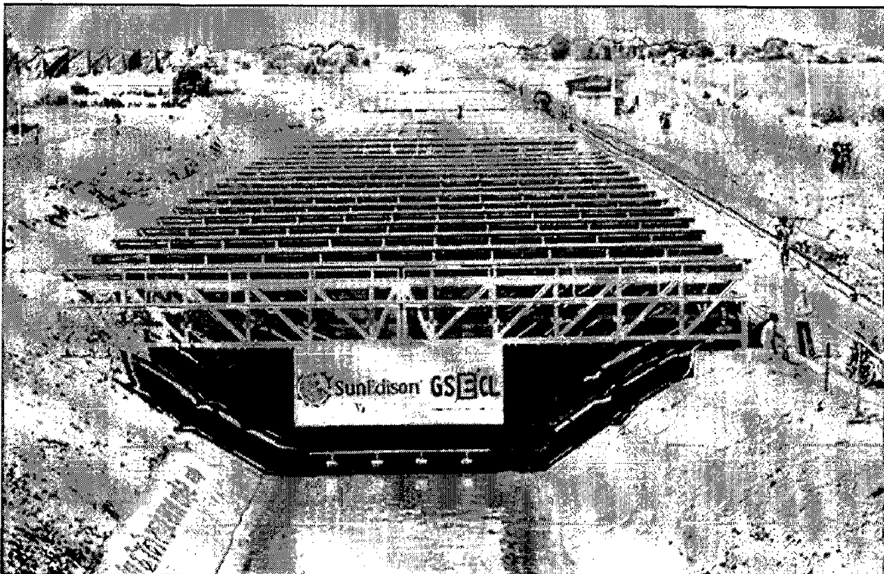
Figure 5-3: solar panel's installation over drains in Gujarat
