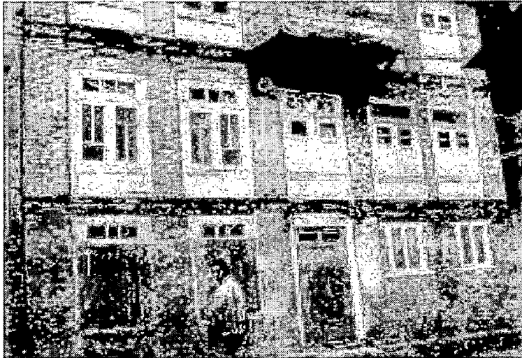
Figure 3.5 Traditional house with Taq construction and corner detail
