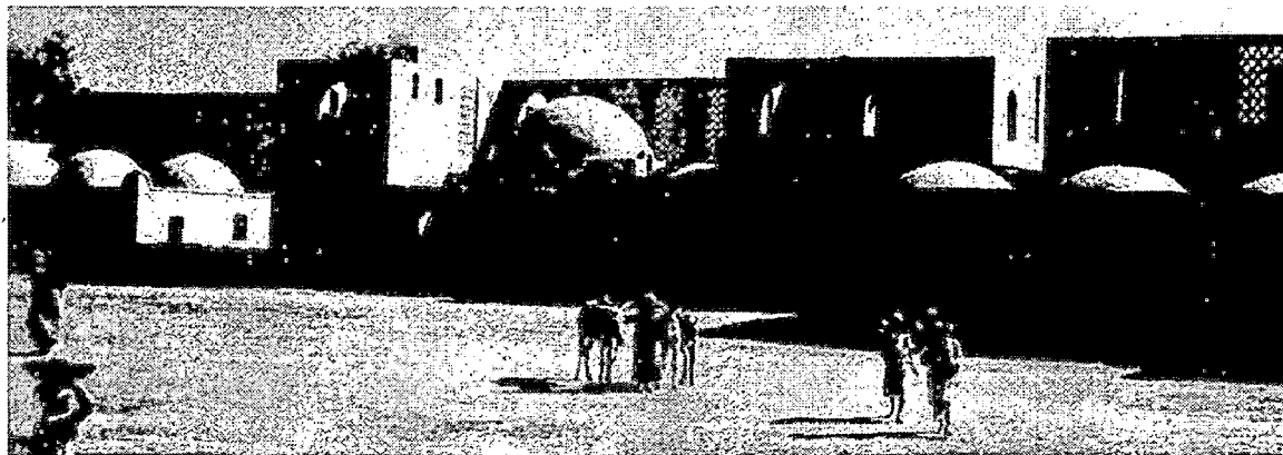
Figure 2.26 Gournah mall: Brilliant use of Vaults and domes
