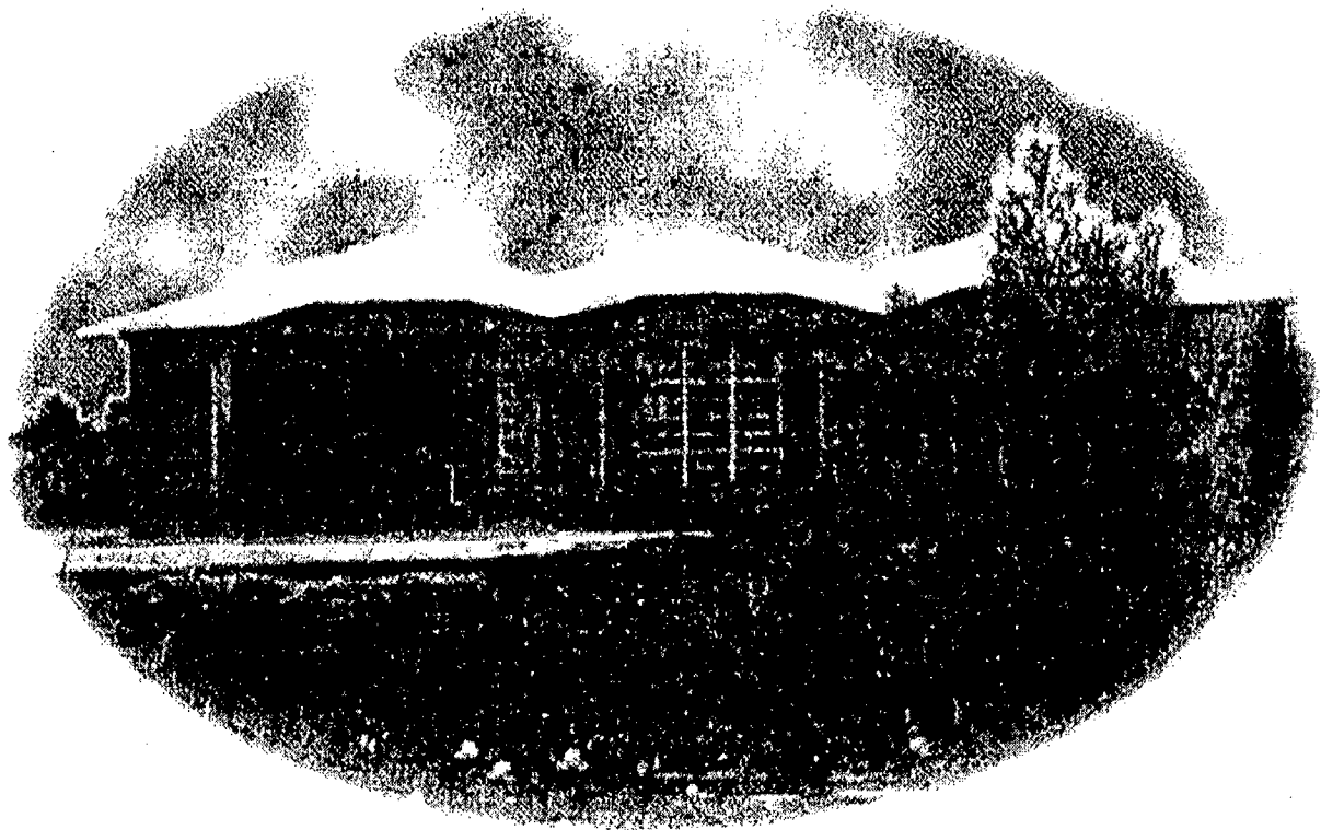
FIGURE 4.5.1: A SOUTH VIEW OF THE HOUSE WITH WINDOWS FOR WINTER GAINS. THE ROOF OVERHANGS PROVIDE SHADING FOR OVERCOMING SUMMER GAINS.
