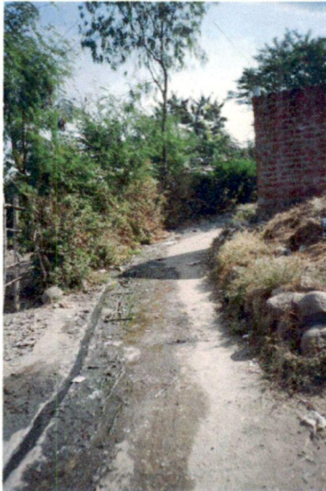
figure 5.5 This figure highlights the ill design and maintenance of open drainage. The agricultural area are heavy users of the water for the purpose of irrigation The isolated residences in the rural area are generally located abutting the field.
