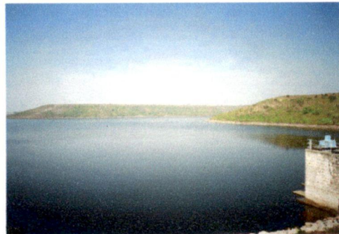
figure 5.20 Kalia sot dam is the source of canal
