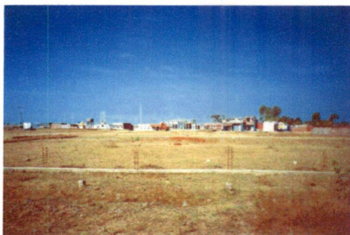
figure 5.7 Large scale construction work being carried in Neelbad village by builders and colonizers.
