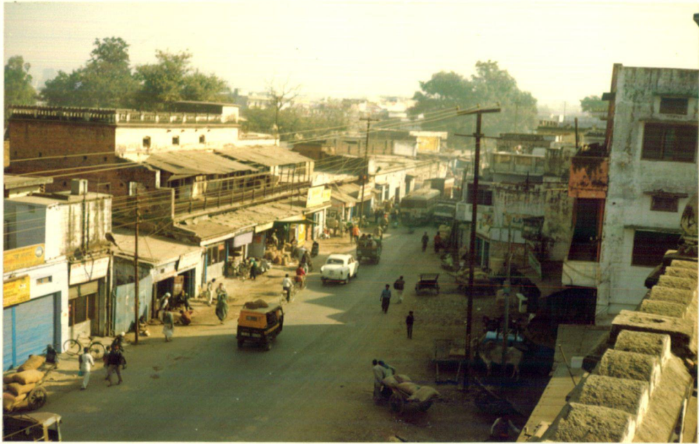
Building Condition in Arat Bazar.
