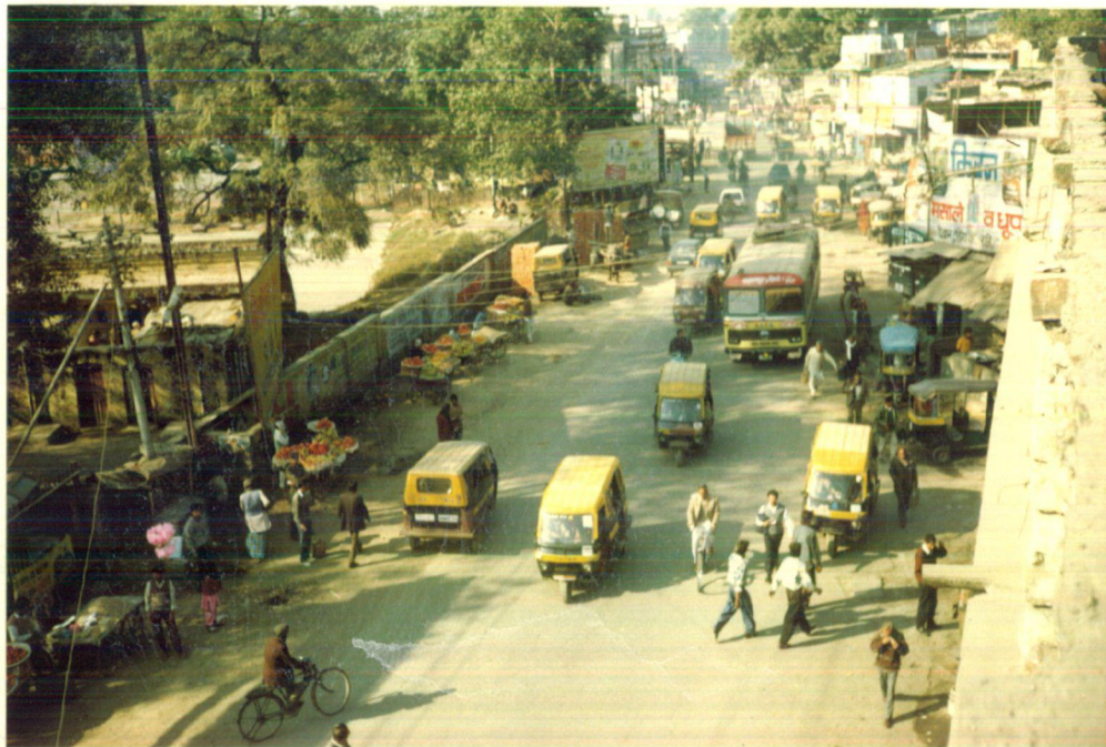
Inadequate Pedestrian path : Opposite lakhibag Police Station
