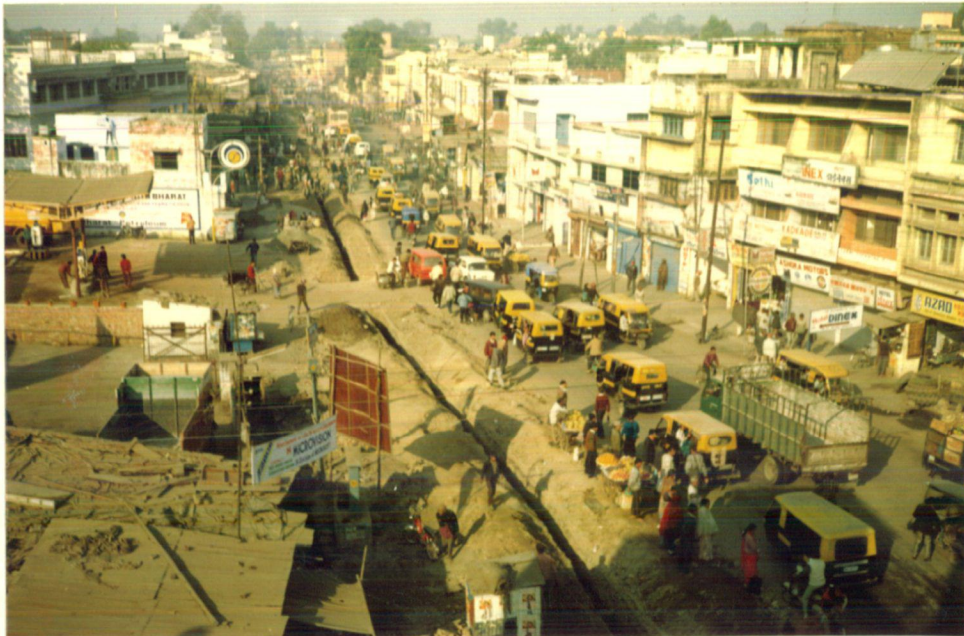
Road side construction work, Improper maintenance, Improper Parking facilities and pedestrian facilities at Prince Hotel Crossing causing visual Pollution
