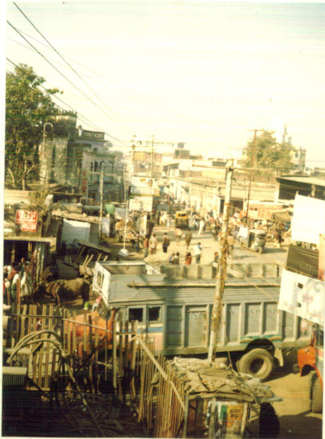
Improper Street Furniture, Bad Condition of building at Arat Bazar.
