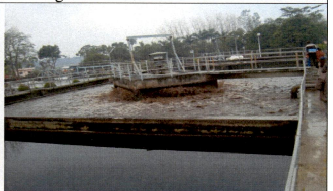
Fig 4.3.4: Aeration Tank
