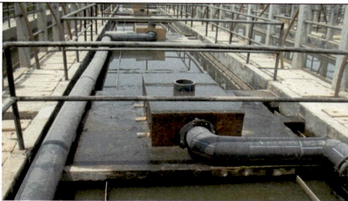
Fig 4.4.3:UASB Reactor
