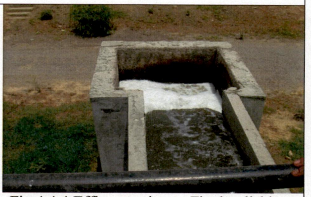
Fig 4.4.4:Effluent going to Final polishing pond
