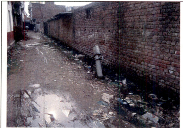
Figure 3.7: Existing situation pumping hand of water supply
