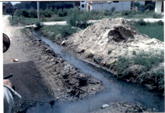
Figure 3.26: Sewage flow is draining through the surface.
