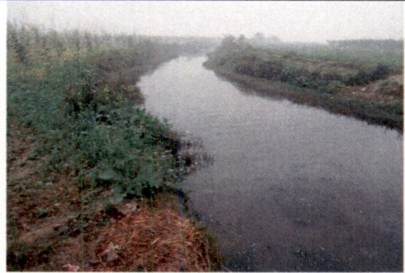
Figure 3.32: Sewer Line (W2)
