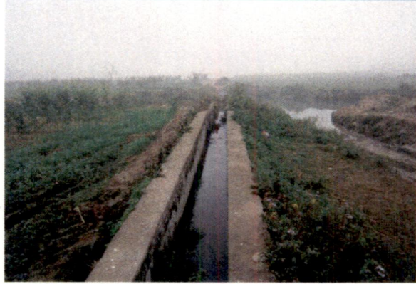
Figure 3.31: Sewer Line (W1)
