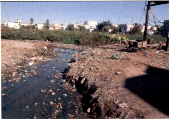
Figure 3.23: Discharge sewer line into sewage pool in the area (1).
