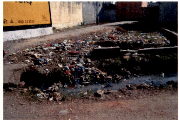
Figure 3.18: Main sewer line from Ramnagar area.
