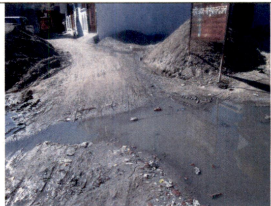
Figure 3.20: Sewage flow is draining through the surface.
