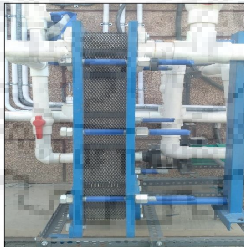
Figure 3.5 Plate heat exchanger
