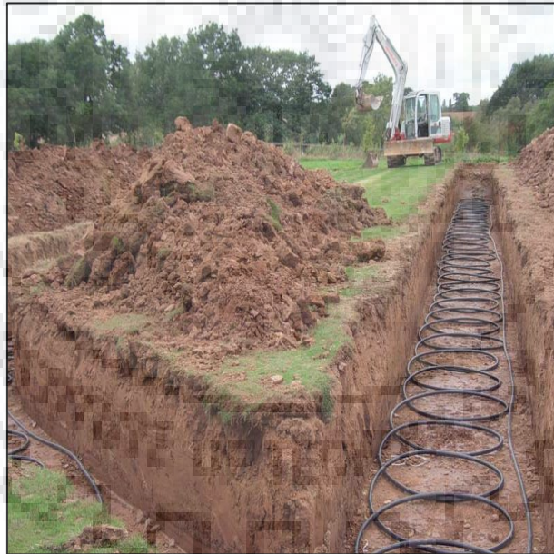
Figure 1.5 Slinky type horizontal GHE
