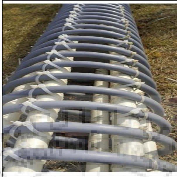
Figure 1.6 Spiral type horizontal GHE (Jeon et al., 2018)
