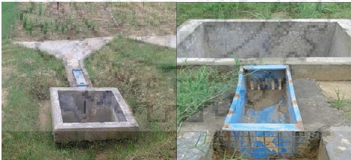
Figure 3.4 Collection Chamber with the multi-slot divisor
