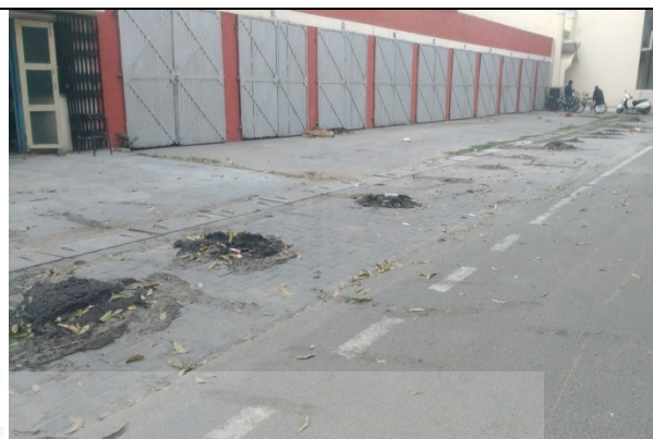
4. Sludge lying aside the road and leads to foul smell
