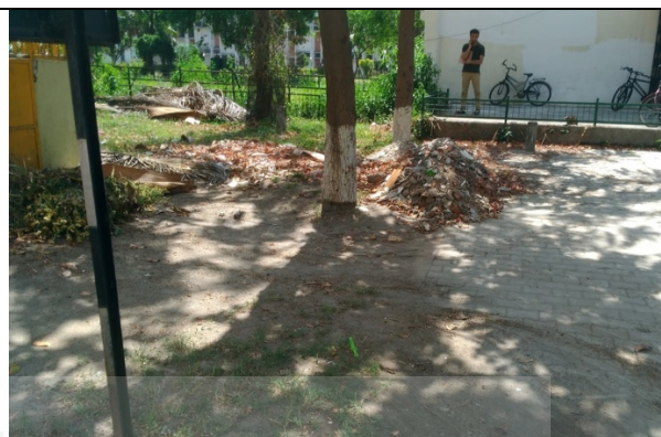
12. After 3 weeks demolished waste was removed
