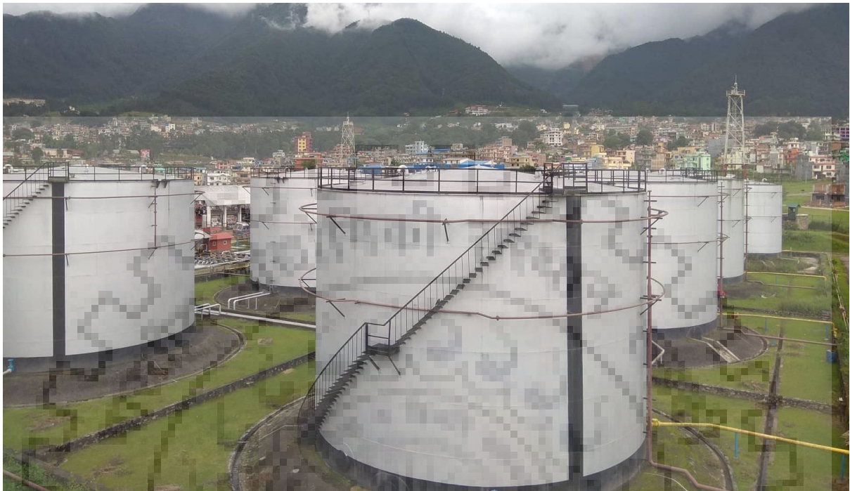
Figure 3.11 Bird's Eye View Image of Fuel Storage Vertical Tank/ Tank Farm Area.
