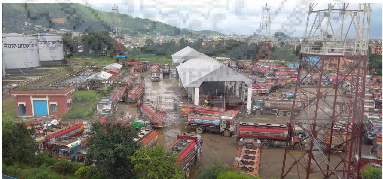
Figure 3.10 Bird's Eye View of Available Rooftop Area of Fuel Tank Truck Loading/Unloading Shed.
