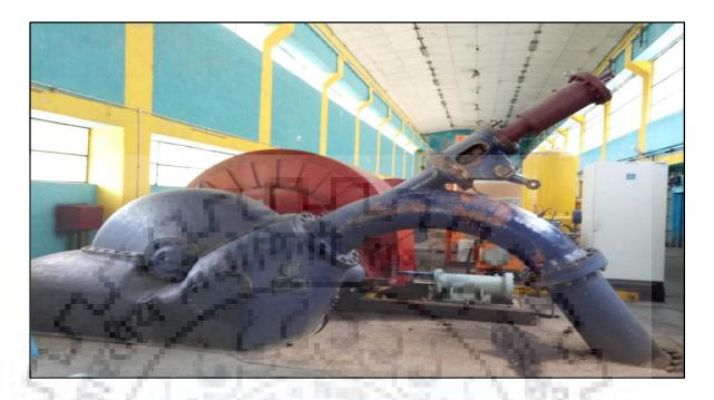
Figure 3.15: Twin jet horizontal shaft Pelton Turbine installed at CHEP-I.
