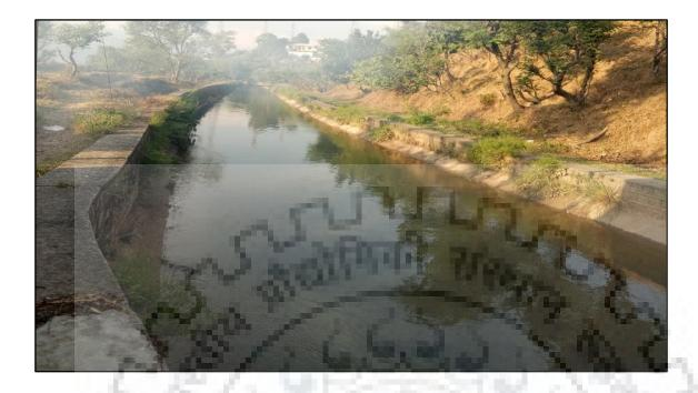
Figure 3.7: Trapezoidal Power channel of CHEP-I.
