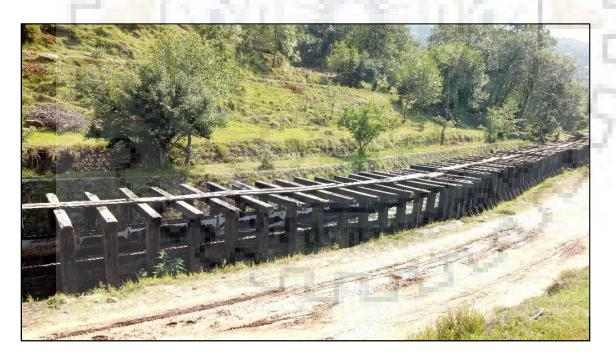
Figure 3.8: Wooden flumes channel of CHEP-I.
