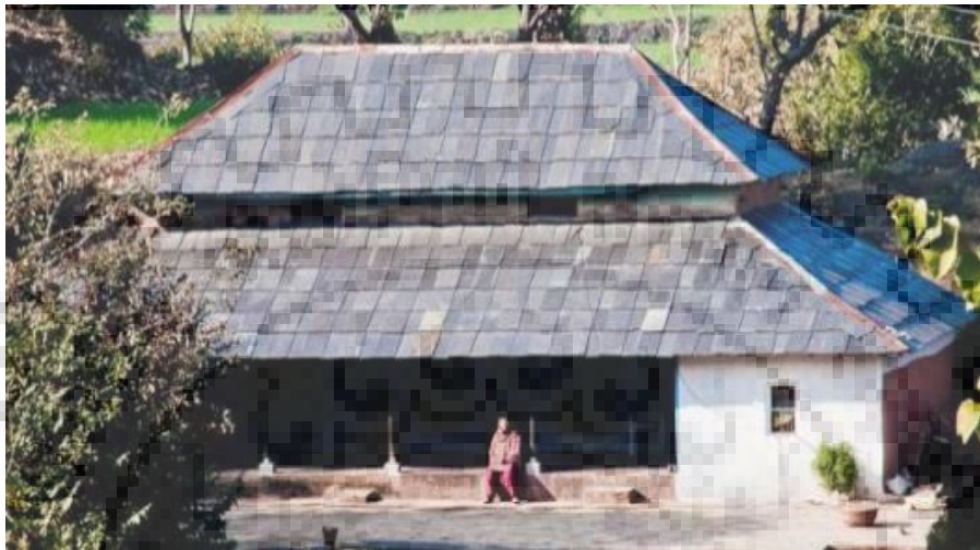
Figure 21 Traditional representative building
