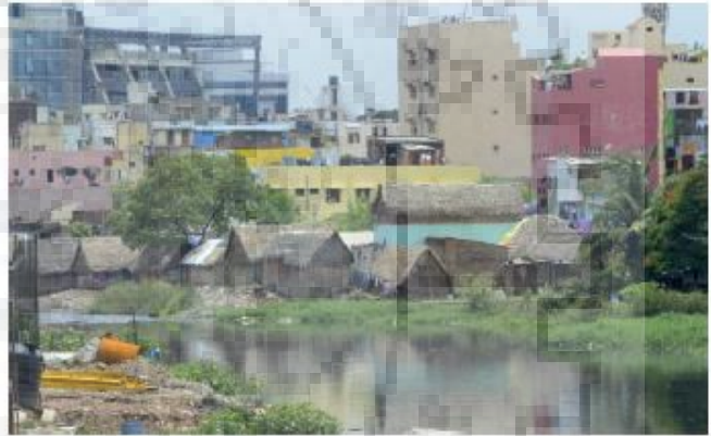
Encroachments along Cooum River
