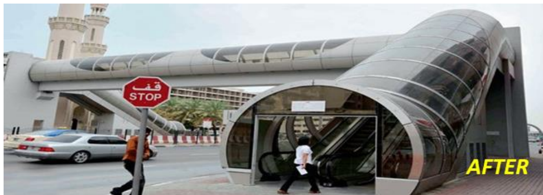
Figure 65 Before and after pictures (Source: Dubai metro)
