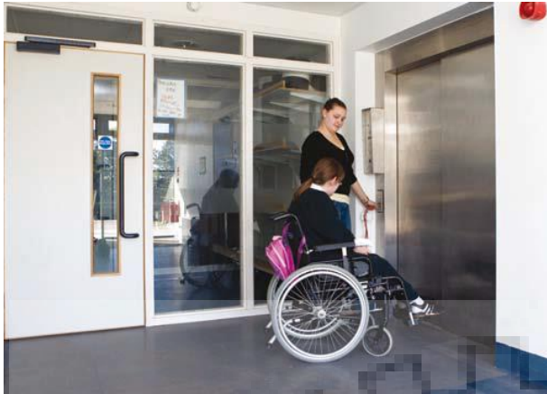
Figure 16 Accessible Lift fitted with Tactile Information
