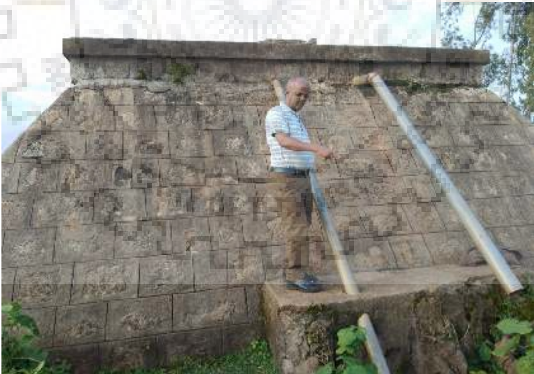
APPENDIX A2 Old masonry tank
