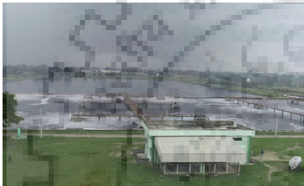
Fig.3.4.2c Aerated Lagoon (Aerobic Process)
