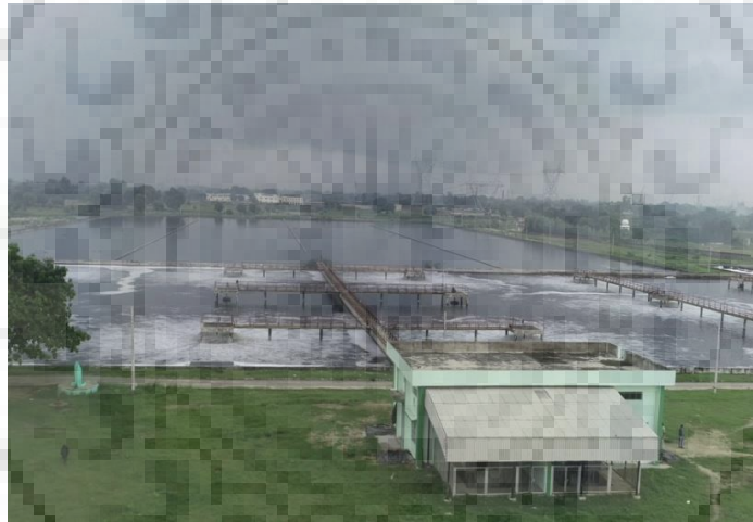
Fig.6.2.2c Surface aerator for aerobic process
