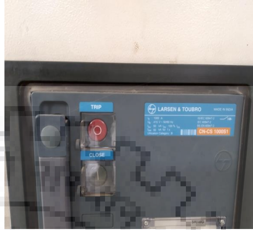
Fig.6.2.2b Starter for filter press belt
