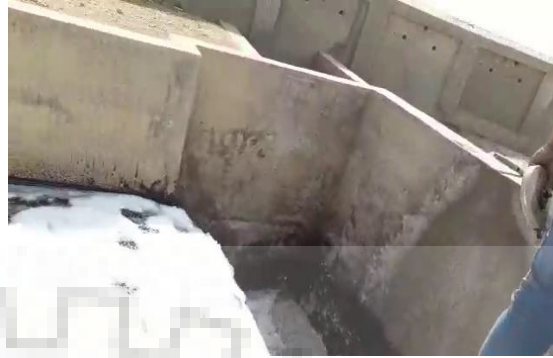
Fig.6.2.1b Drop at the end of outlet channel
