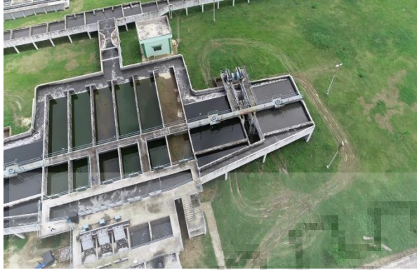
Fig.3.4.2a Screening and Grit Chamber
