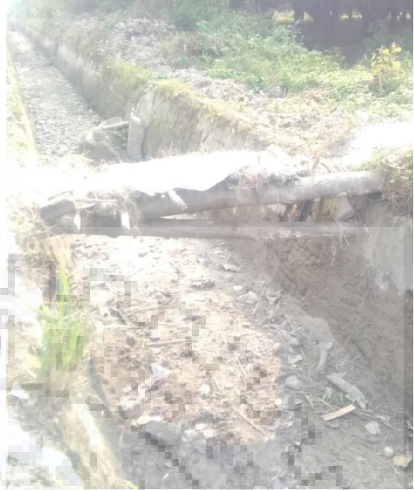
Photo 5.10 Temporary foot bridge
