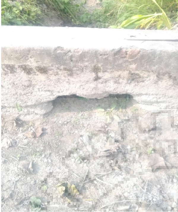
Photo 5.9 Damaged outlet
