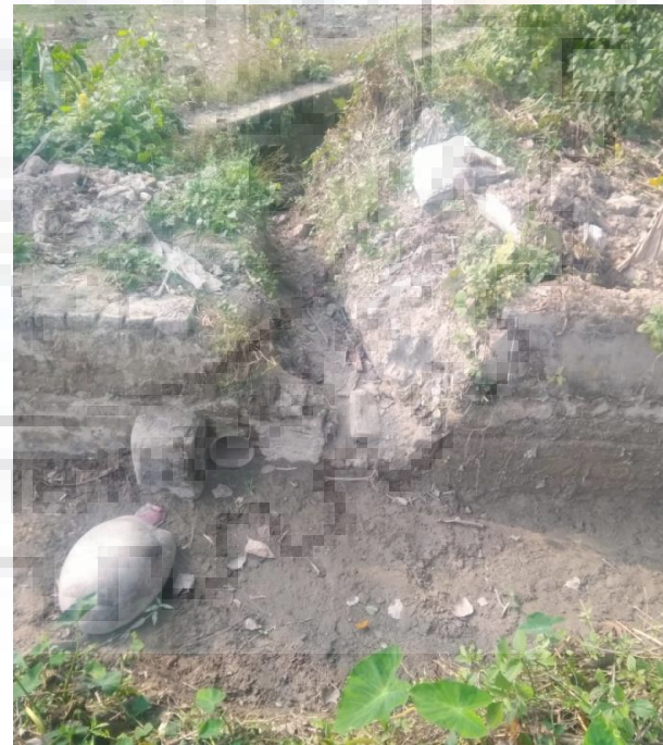
Photo 5.8 Canal bank cutting to draw more water
