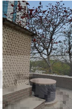
Figure 59 Light wells on roof
