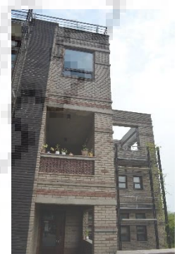
Figure 57 Balcony attached to each floor
