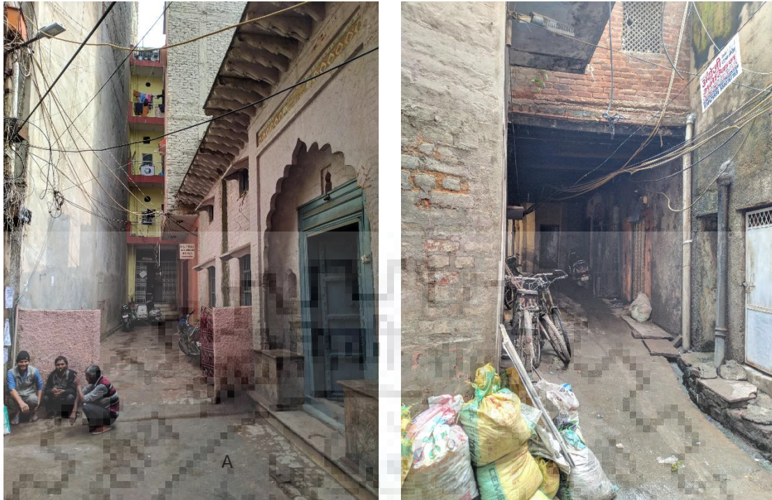
Figure 52 Dead end street encroached by residents with boundary walls and cantilevers
