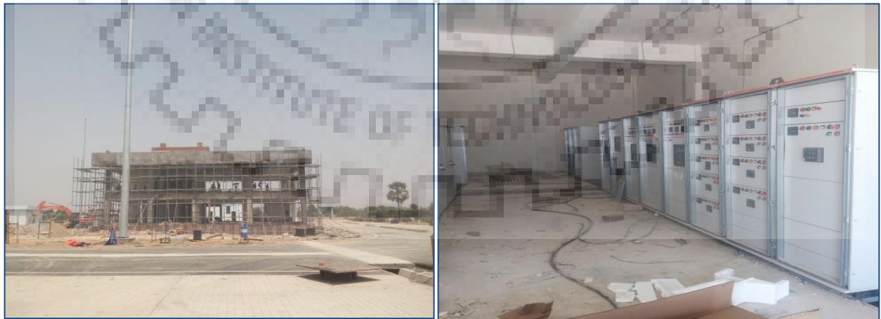
Figure 21: Ongoing construction work at Varanasi inland waterway terminal
